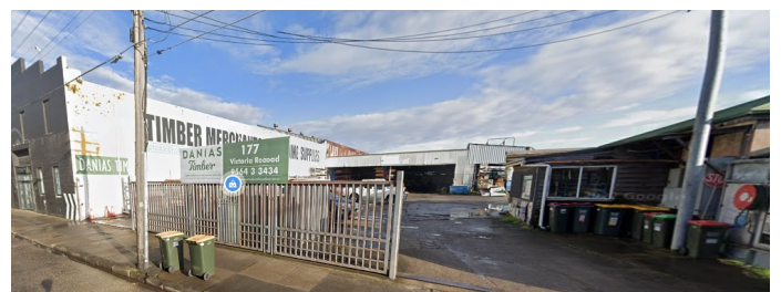
Danias Timberyard (Photo: courtesy of Google, 2022)
