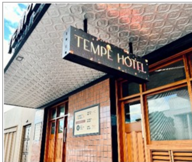
Detail – revamped façade of the Tempe Hotel (Courtesy Tempe Hotel website)
