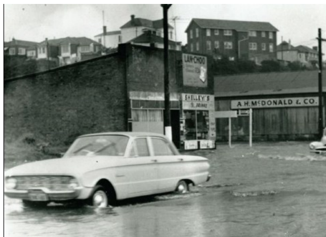
Illawarra Road, Marrickville in flood near Wharf Street, probably in the 1960s (Source: Daily Telegraph site)
