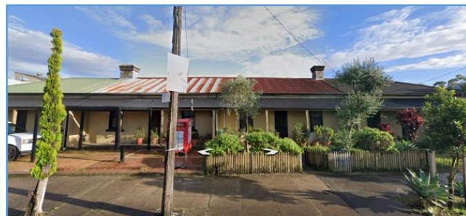
The original 1880s cottages, recently demolished (Courtesy Google)
